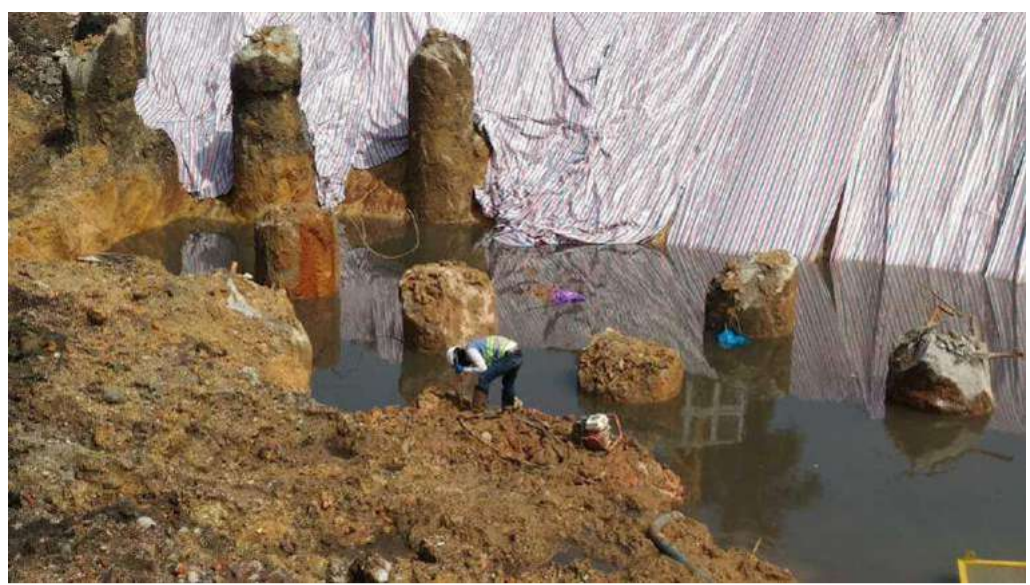
I supervise and check surveyor do as-built for bored pile.
