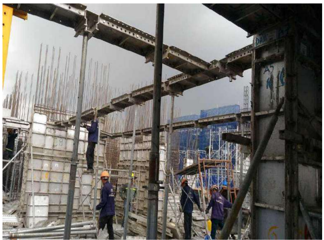
Installing aluminum formwork
