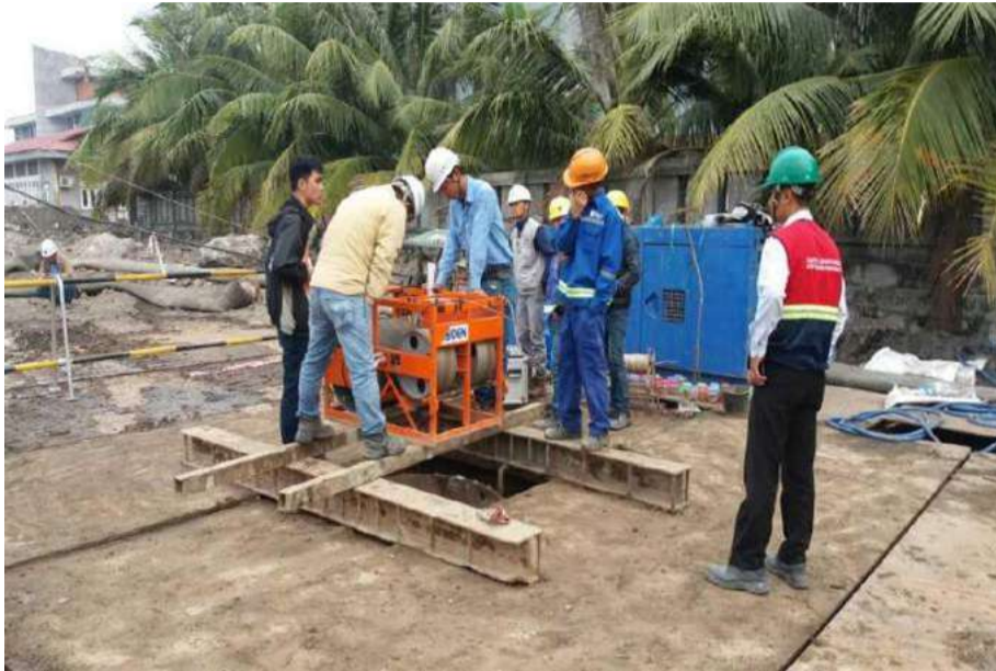
Many engineers are preparing for KoDen testing.
