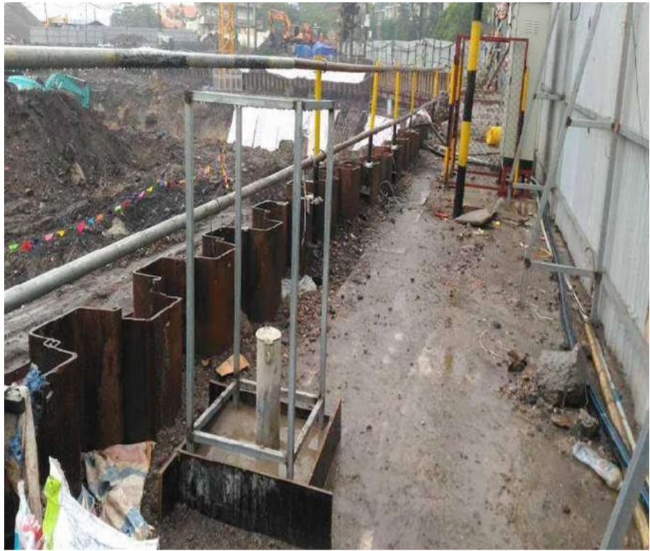
I am QC inclinometer and metal sheet pile and other suveys.
