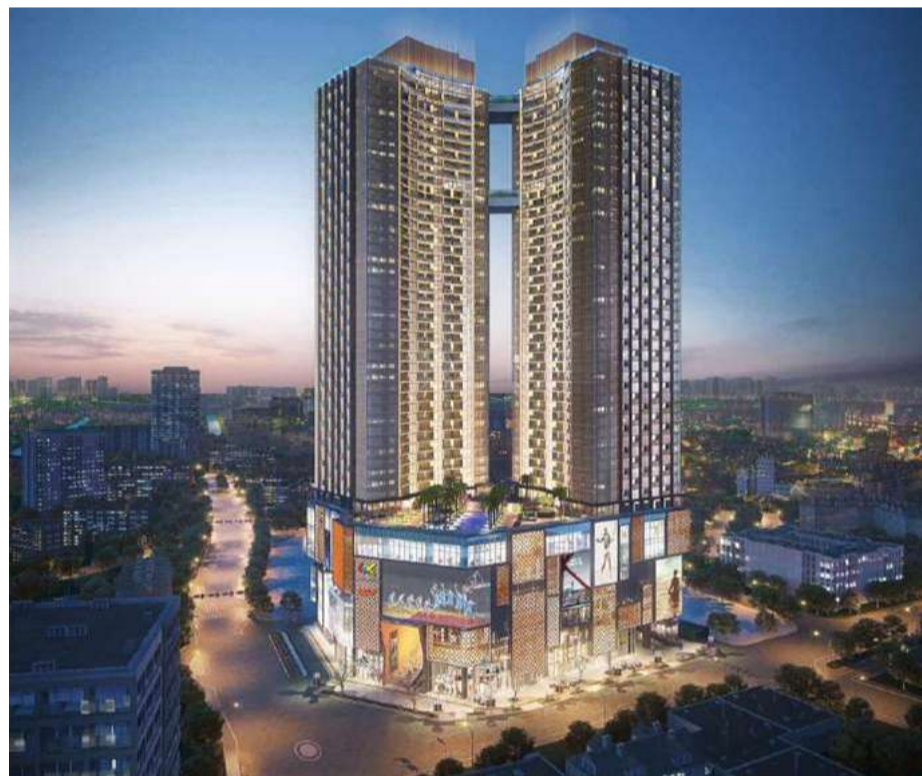
Perspective of project.It cost $ 160 million - 51 floors 4 basements .We bid it.
